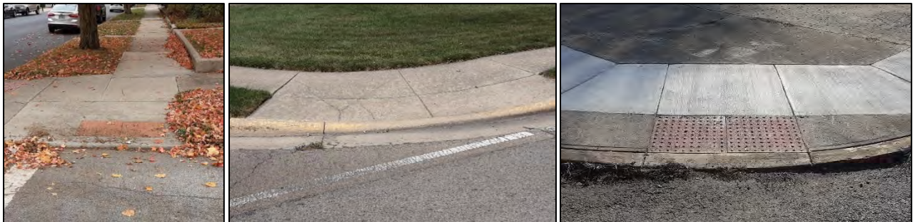
Examples of curb ramps with vertical discontinuities that exceed 1/2" at the curb, on the ramp, or the TS.
