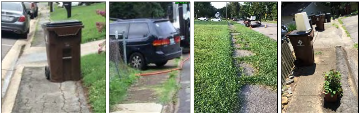
Examples of temporary obstructions of the PAR that reduce the width to less than 48" (note these are not actual photographs in the City).
