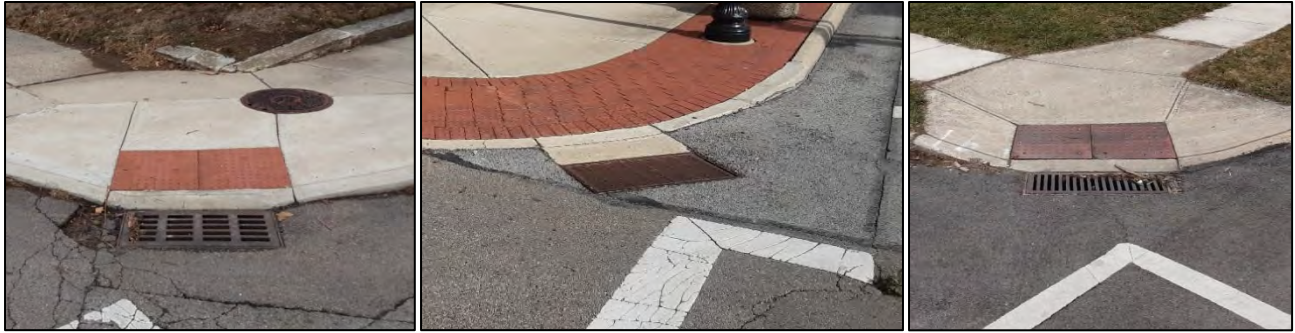
Examples of curb ramps with utility structures on the ramp or the clear space.
