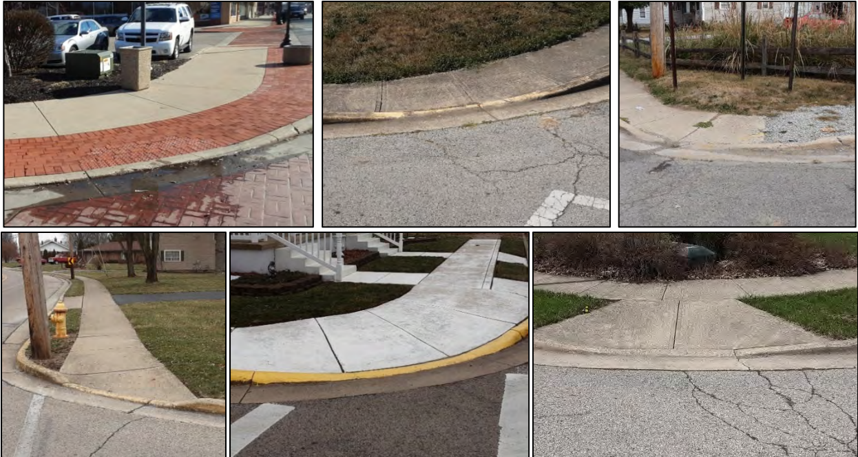
Curb ramps lacking DWs as required or which have low contrast.
