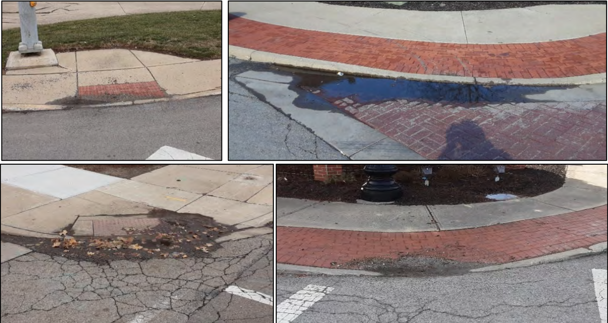
Examples of curb ramps with drainage issues and/or evidence of regular ponding, with sediment deposition.
