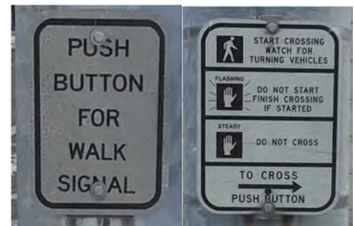
Example of non-compliant signage that includes only visual text and fully compliant sign with text, arrow, instructions, and pictograms.
