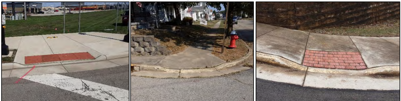
Example of curb ramps that have non-compliant flare slopes.
