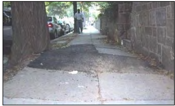
Temporary patching for large displacements
