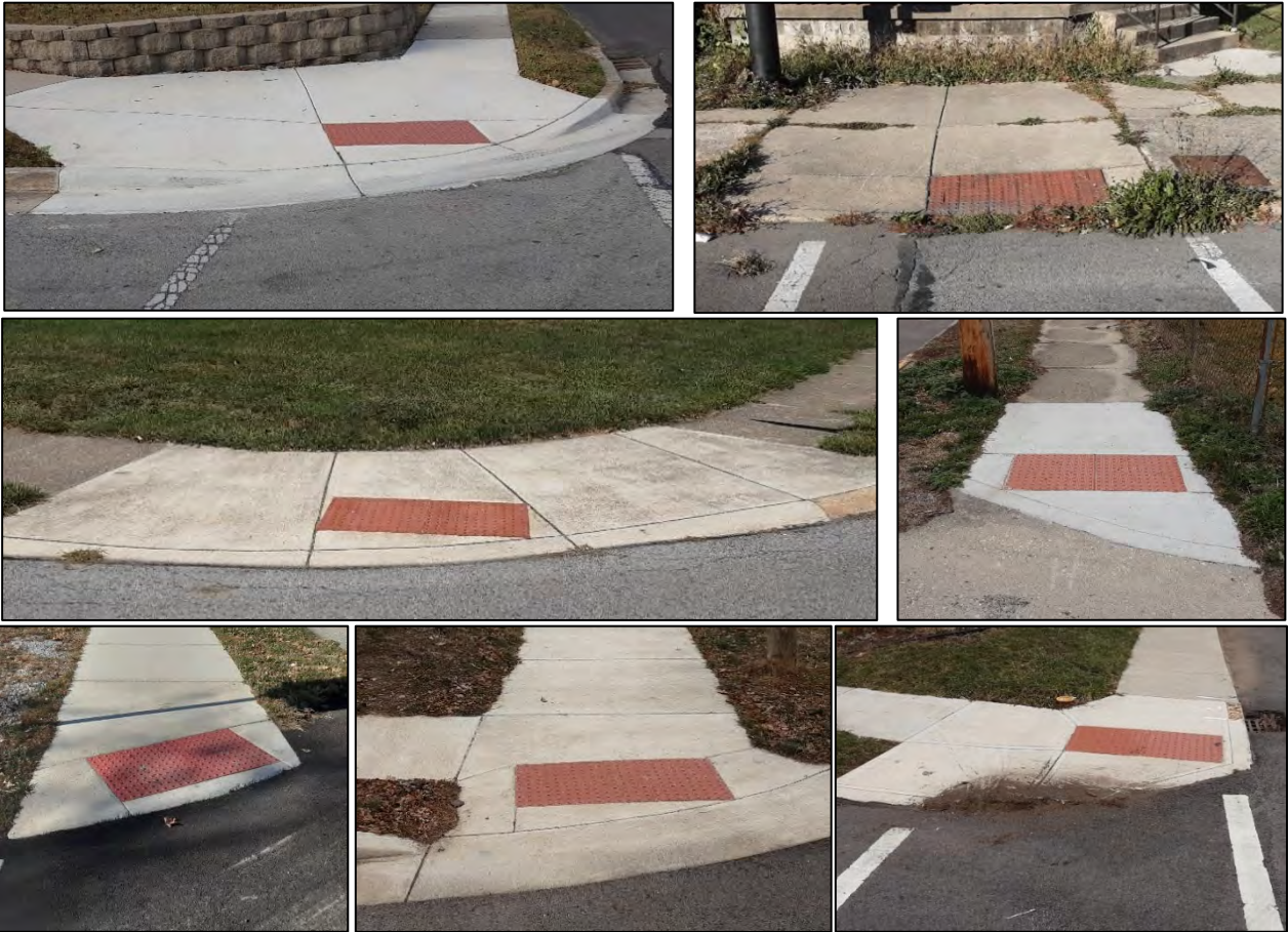
Example of curb ramps with detectable warnings that are not full width of the ramp.
