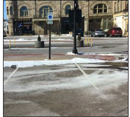
Accessible on-street parking space with no access aisle.
