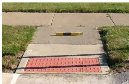
Examples of typical perpendicular curb ramps, with and without flares based on presence/absence of PCA.
