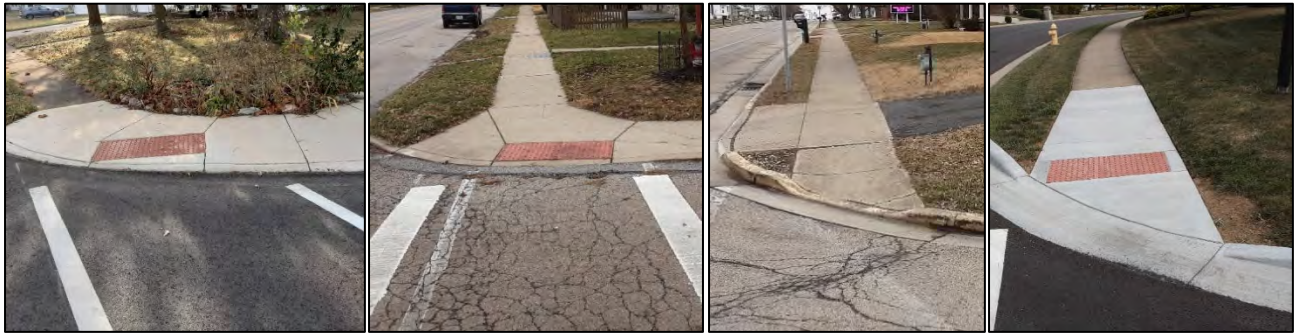
Curb ramps with excessive cross slopes. These ramps also typically have non-compliant landing cross slope.
