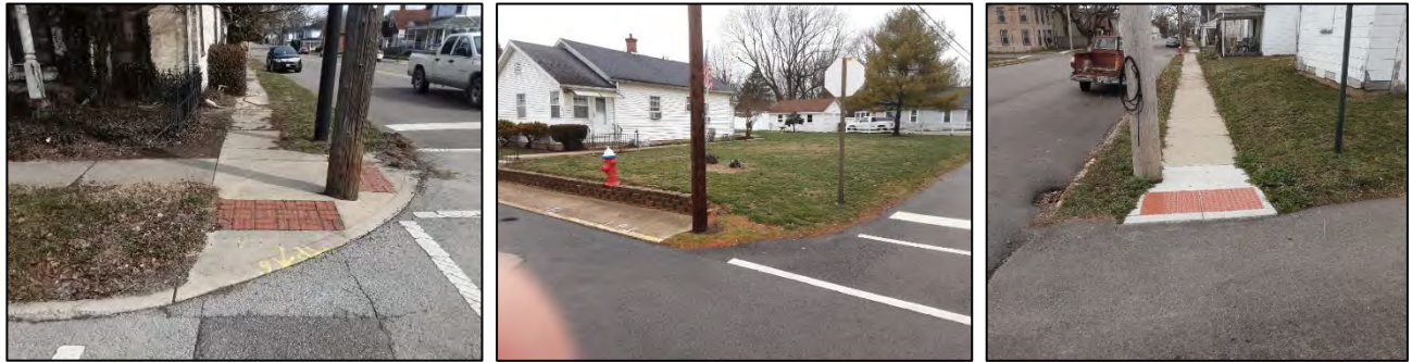
Examples of curb ramps with obstructions at turning spaces, on the ramp, or immediately adjacent to either.
