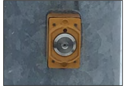
Example of typical pushbutton that is 2" diameter but includes no tactile directional arrow on the pushbutton.
