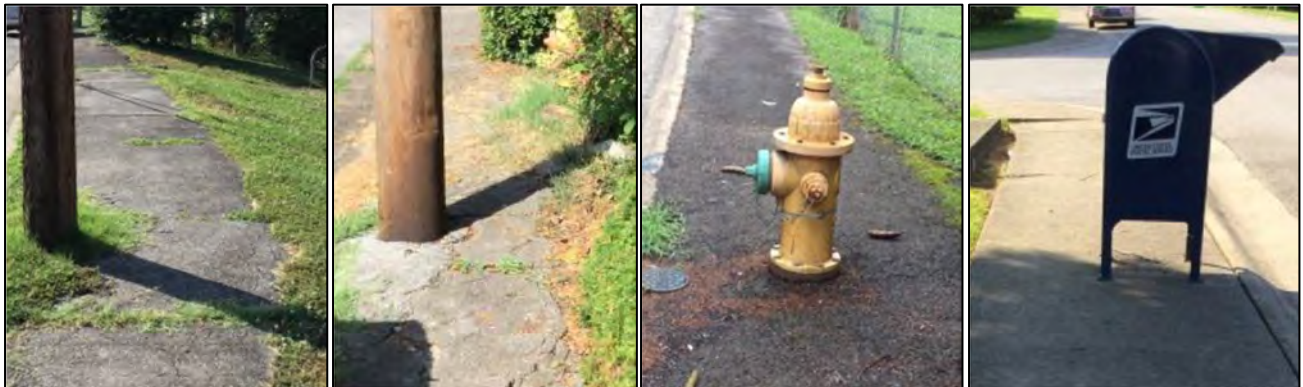
Examples of more permanent obstructions of the PAR that reduce the width to less than 48" (note these are not actual photographs in the City).
