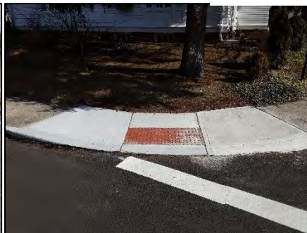
Example of curb ramps that have no clear space or clear space is not within crosswalk.
