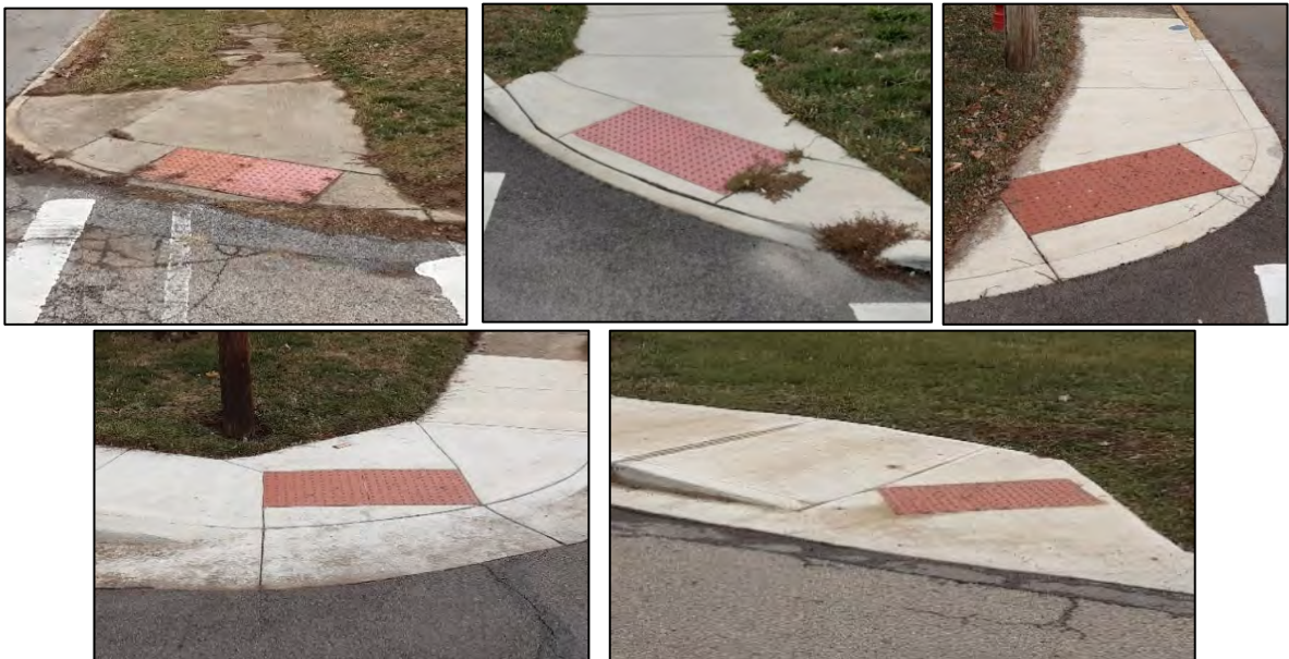
DWs that are oriented poorly and are not 24" depth in entire direction of pedestrian movement.
