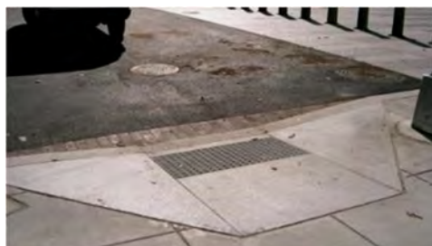
Examples of typical perpendicular curb ramps, with and without flares based on presence/absence of PCA.
