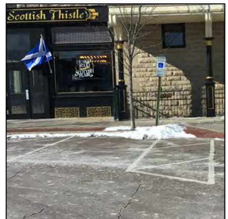
Accessible on-street parking space with non-compliant width access aisle.
