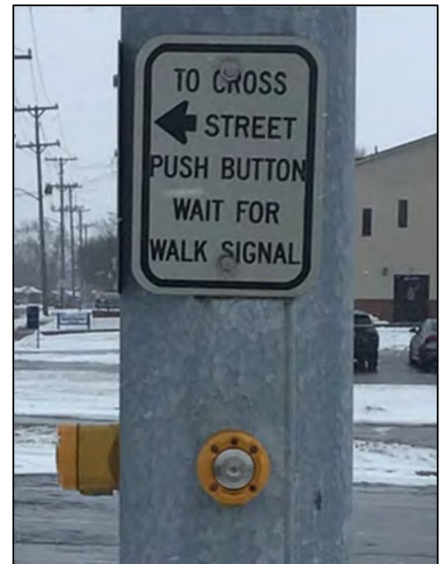
Example of pushbuttons on shared pole with sign that includes visual text and arrow indicating the crossing direction controlled.
