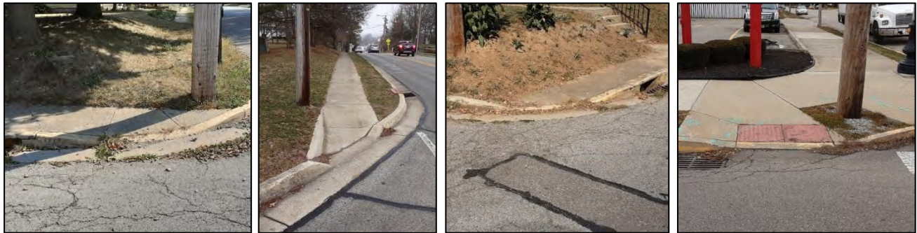
Examples of curb ramps that are less than the minimum 48" width required.
