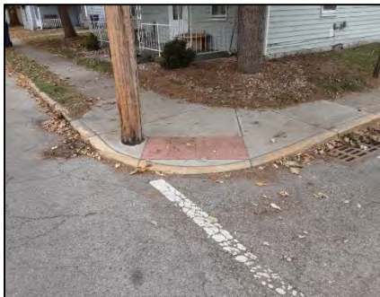
Example of curb ramps that have no clear space or clear space is not within crosswalk.
